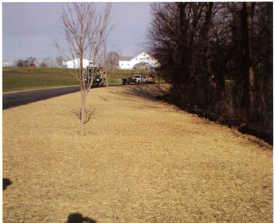
Rapho Township in Lancaster County relocated a road when replacing a bridge damaged by Tropical Storm Lee in 2011. The road originally ran along a stand of trees (top), with a creek just on the other side of the trees. During the reconstruction, the township moved the road about 50 feet away from the trees so that it is out of the direct floodway (bottom). (Photos courtesy of Rapho Township.)
